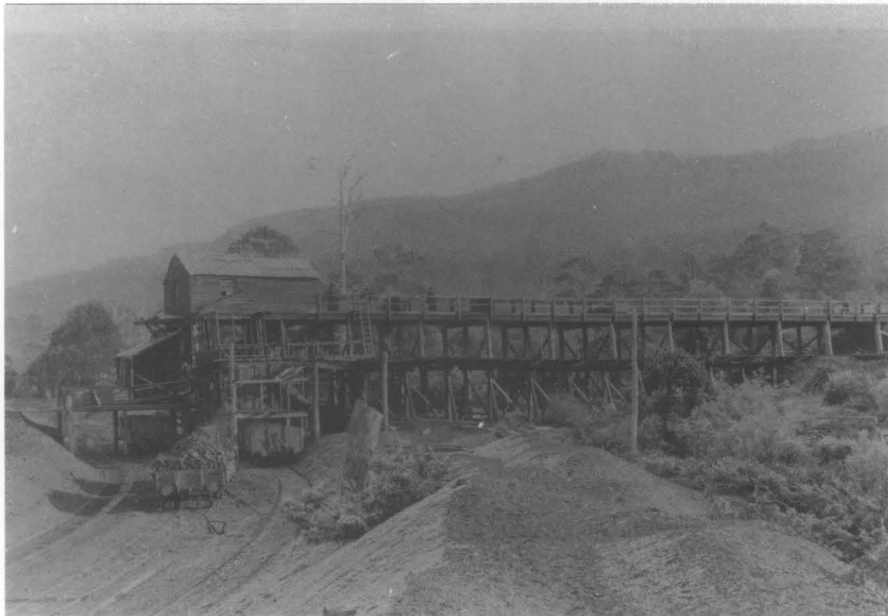
After mining the coal was conveyed via a self-acting tramway to loading bins above the railway siding at Cullenswood. The bins at this location were rebuilt and expanded over the years, and served as the main loading point until the closure of the mine. Current output from the Cornwall area is trucked to Fingal for washing and loading. [Cornwall Coal]
