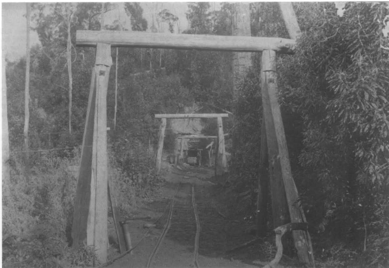
Entrance to the main heading on the Cornwall Seam, circa 1904, showing cable for hauling loaded skips. [Cornwall Coal]
