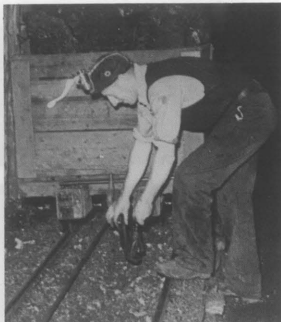
Attaching loaded skips to the winding cable, Cornwall Mine. (above)
