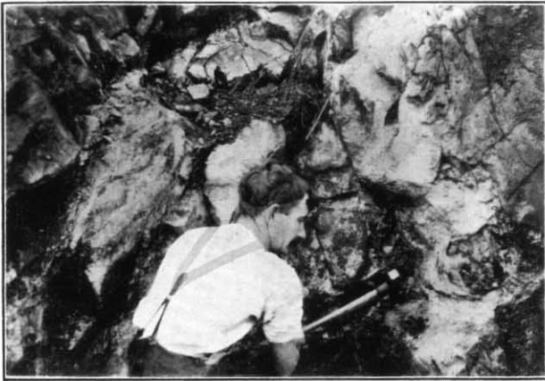
Quarrying Solid Serpentine Rock for Osmiridium, Bald Hill.
