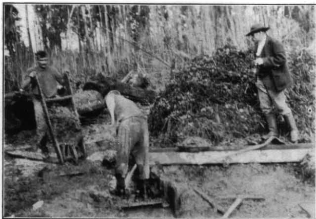
Sluicing Mud for Metal at Wilson River.
