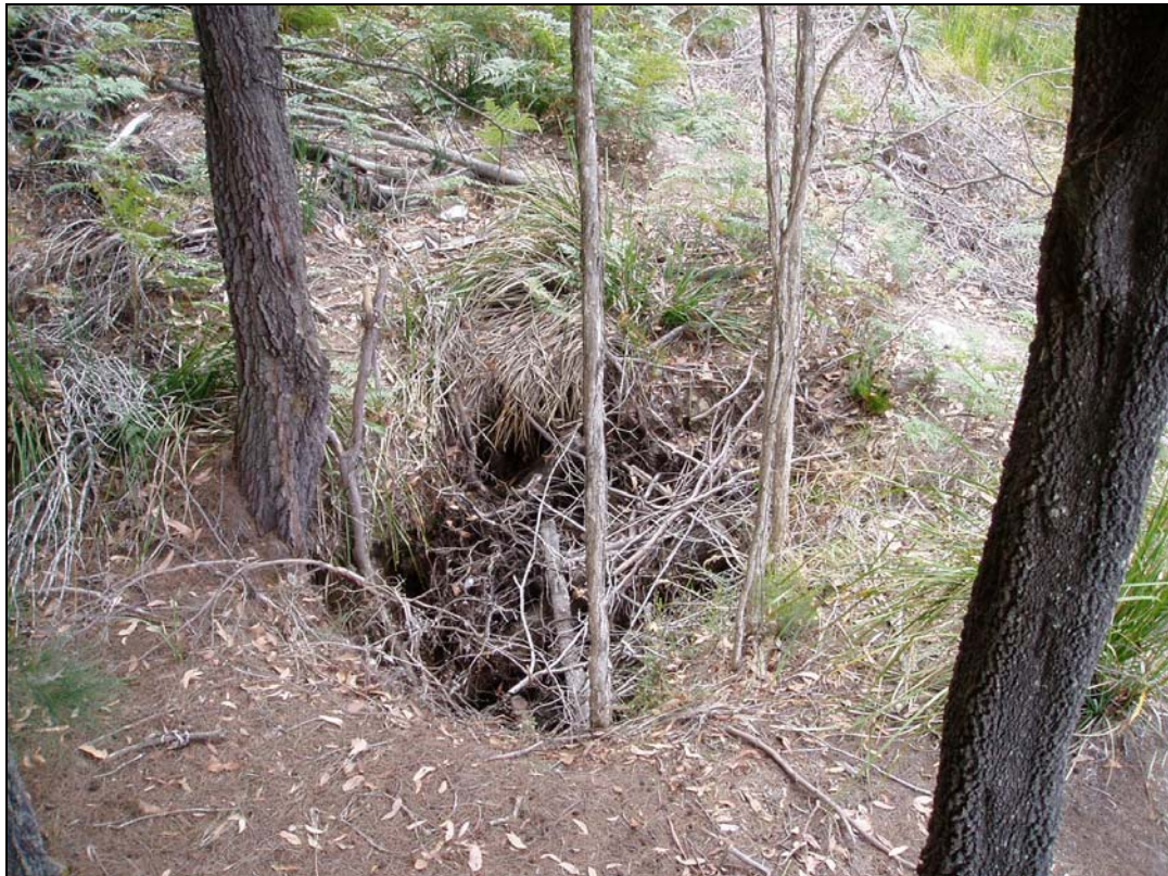
Figure 4. Shaft on Golden Era line, 2500 mm x 2000 mm and open to 8 metres.
