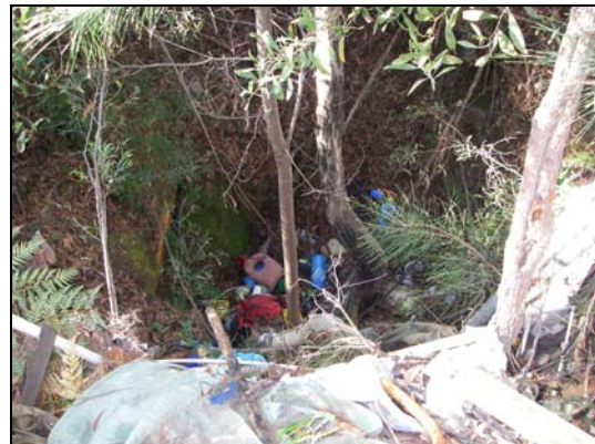
Figure 7. Reward Main Shaft. The collapse is approximately 10 metres diameter and 8 metres depth to rubbish.
