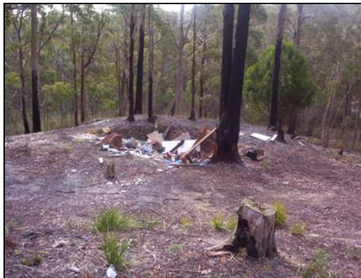
Figure 6. Volunteer shaft. The collapse is approximately 10 metres diameter. Anecdotal evidence is that rubbish is supported by two car bodies wedged into the shaft.
