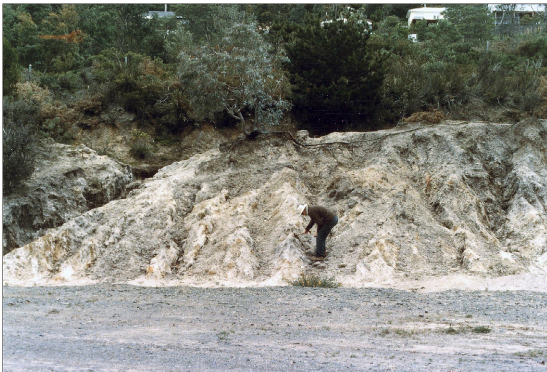
Plate 6. Erosion of exposed banks and cuttings in soils on Triassic sediments — Wellesley Park, South Hobart
