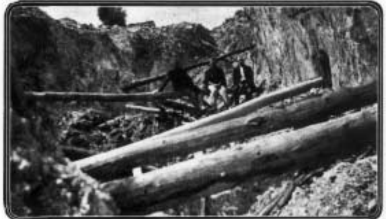
The new lode opened to 30ft. width and heavily timbered. Left to right: Messrs. M. J. O'Reilly, H. Hill (working for Ivory Bros.), and J. Harrison, a well-known identity from the Savage River.
