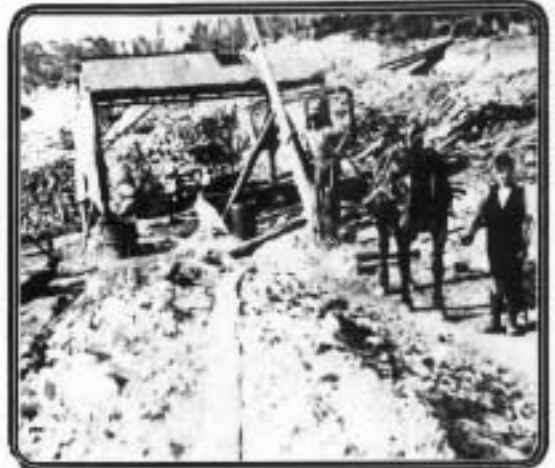
The main shaft on Ivory Bros.' claim. Horse operated "whip" haulage brings lode material to the surface.
