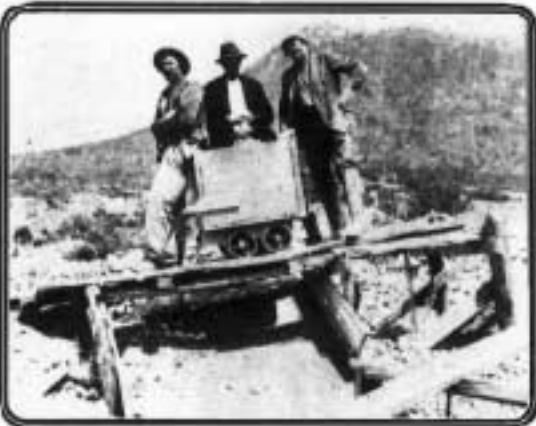
Trucked are at the bin tip to gravitate to tail race, where Falls Creek water at nozzle pressure will sift the sup. Left to right: Messrs. H. Hill, J. Harrison, M. J. O'Reilly.
