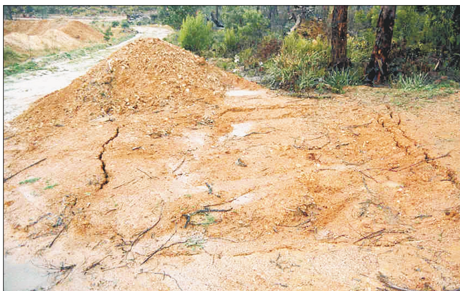
Plate 2. Cracking and slumping of cover material used on a recent pesticide/herbicide/weedicide container burial trench.
