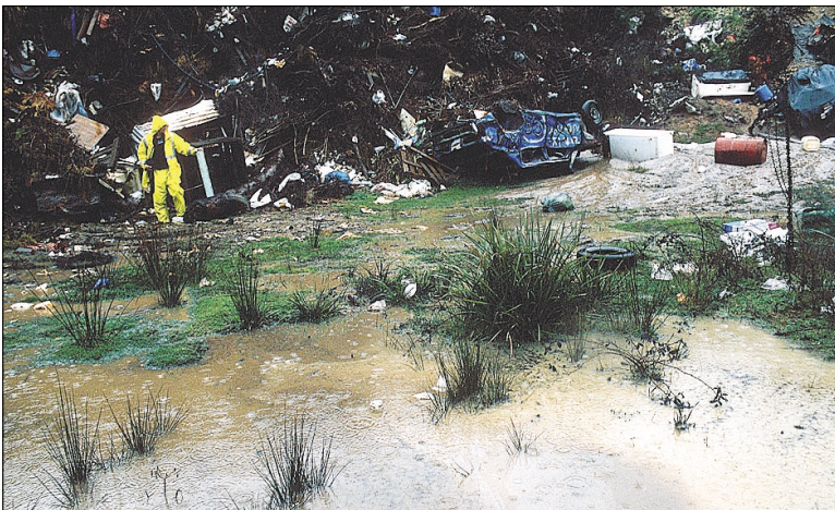
Plate 4. Leachate discharging from the landfill as a spring in a bund wall.
