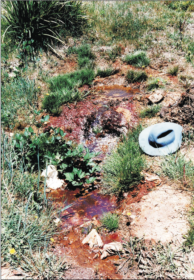
Plate 4. Leachate discharging from the landfill as a spring in a bund wall.
