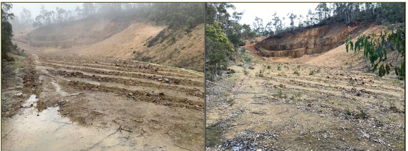
Figure 13. Comparison of Lake River Rd. Quarry indicating establishment of vegetation in rip lines.
