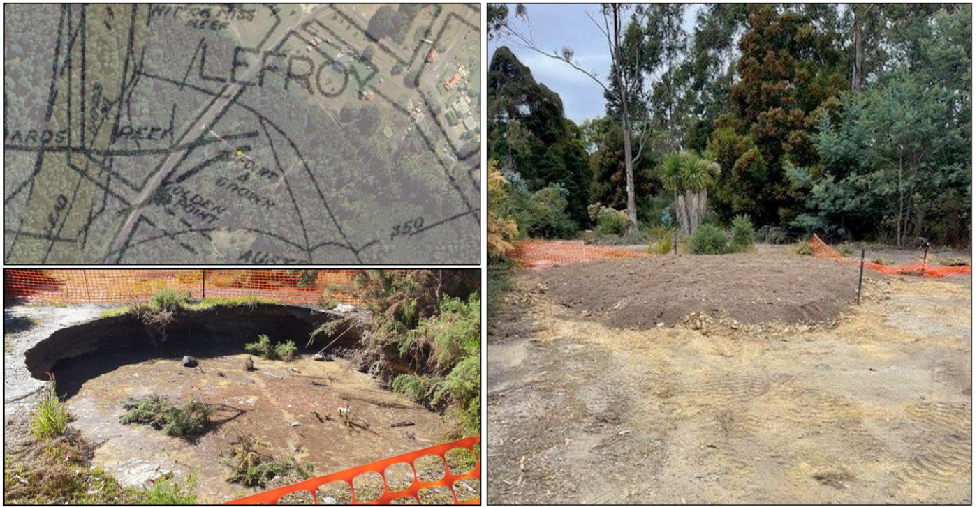
Figure 9. Historical workings overlay (top left), sinkhole (bottom left), and remediation works (right), Lefroy, 2024/25.
