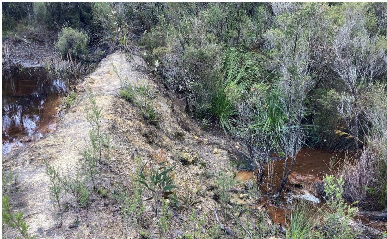
Figure 4. Current condition of Balfour Central Shaft Dam embankment (November 2025).
