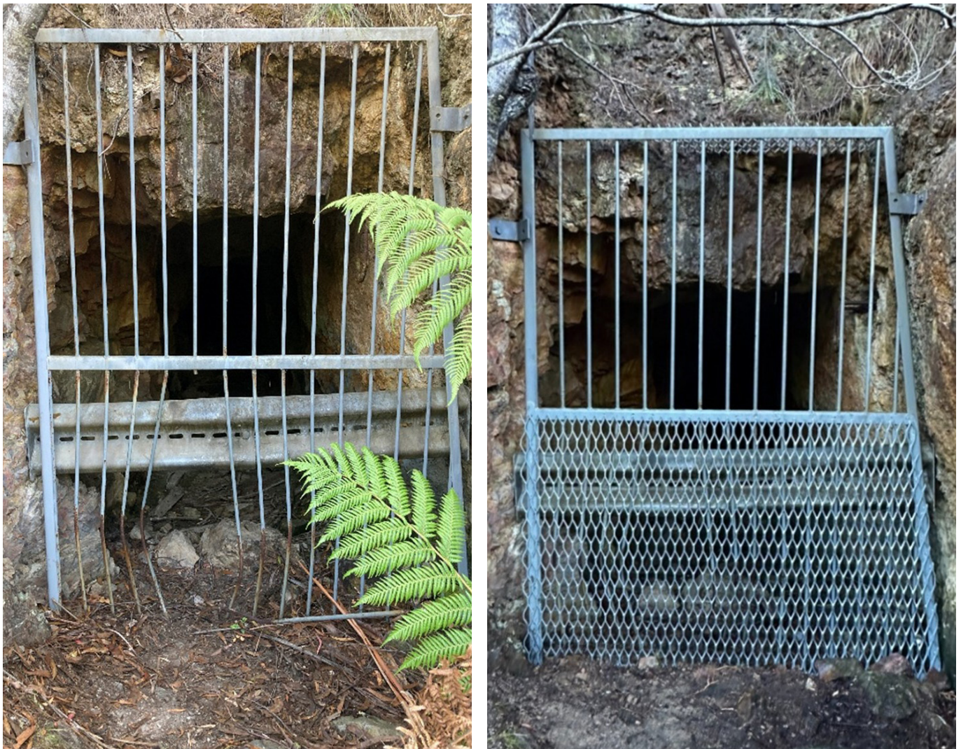
Figure 26. Orieco adit site pre (January 2026) and post repair (April 2026).
