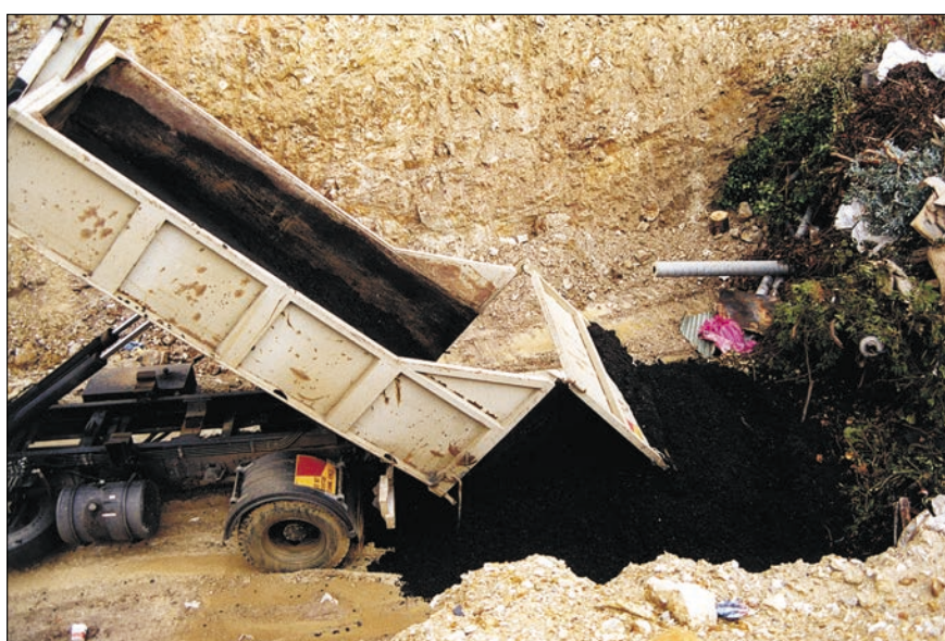
Plate 3 Back filling the western stormwater drain on 17 May 2001.
