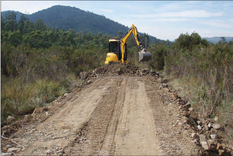
Track construction through buttongrass on peat — coarse fill from local borrow pit.
