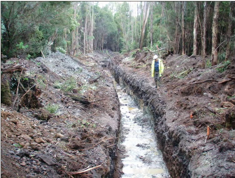
Costean at Stanley Reward showing topsoil to right and gravel to left.
