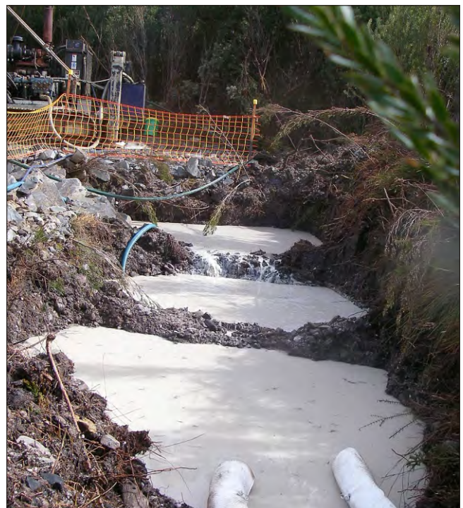
Creek contamination from drill water.
