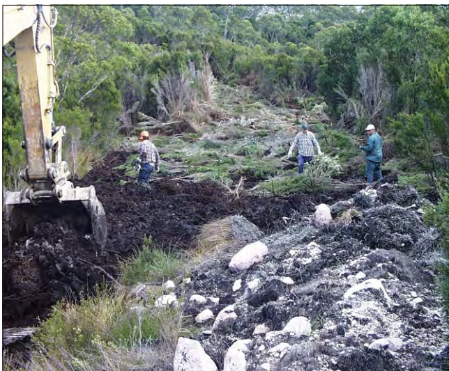
Spreading tea tree slash on drill access track.
