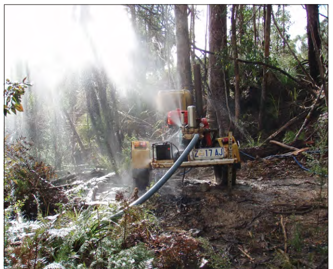
Water spraying from pump and fuel tank with no bund — very poor practice.
