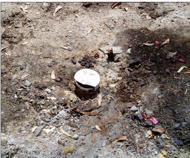
Broken PVC cap on steel collar.
