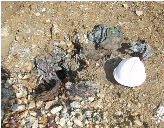
Open hole jammed with grease-soaked rags.
