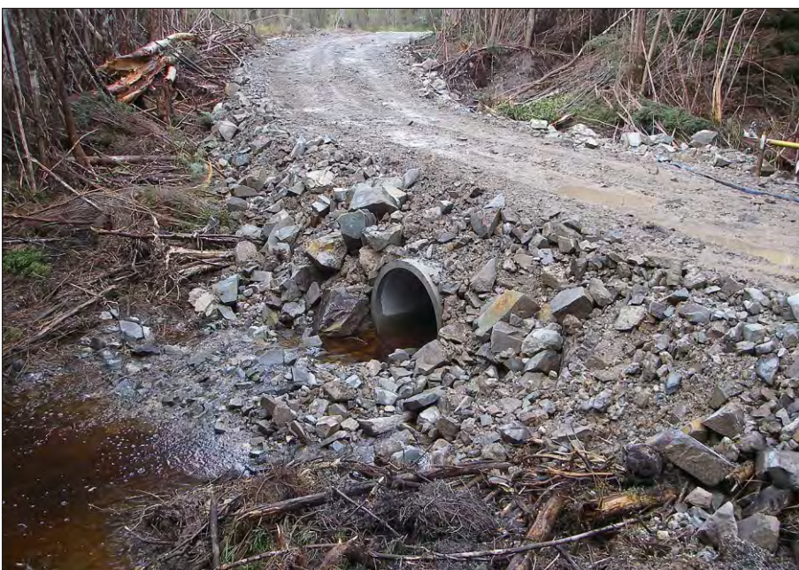
Well constructed concrete pipe culvert.
