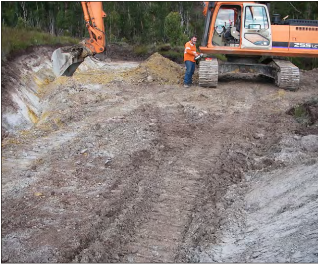
Drill site preparation — note drainage on top side of the pad.
