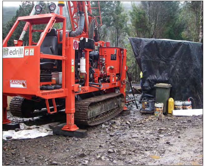
Drill site. Note oil absorbent matting under the rig.
