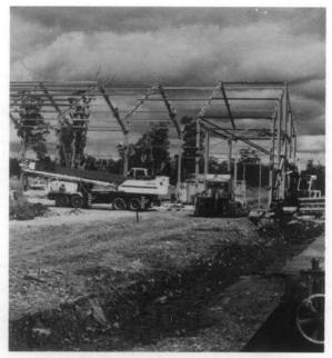
Concentrate storage and loading shed under construction at Hatfield Siding as part of the expansion of production at the Hellyer mine.
