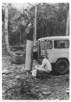
Technician Rohan Sedgman installing a data logger for monitoring roof collapse at the Duncan Mine on Fingal Tier.
