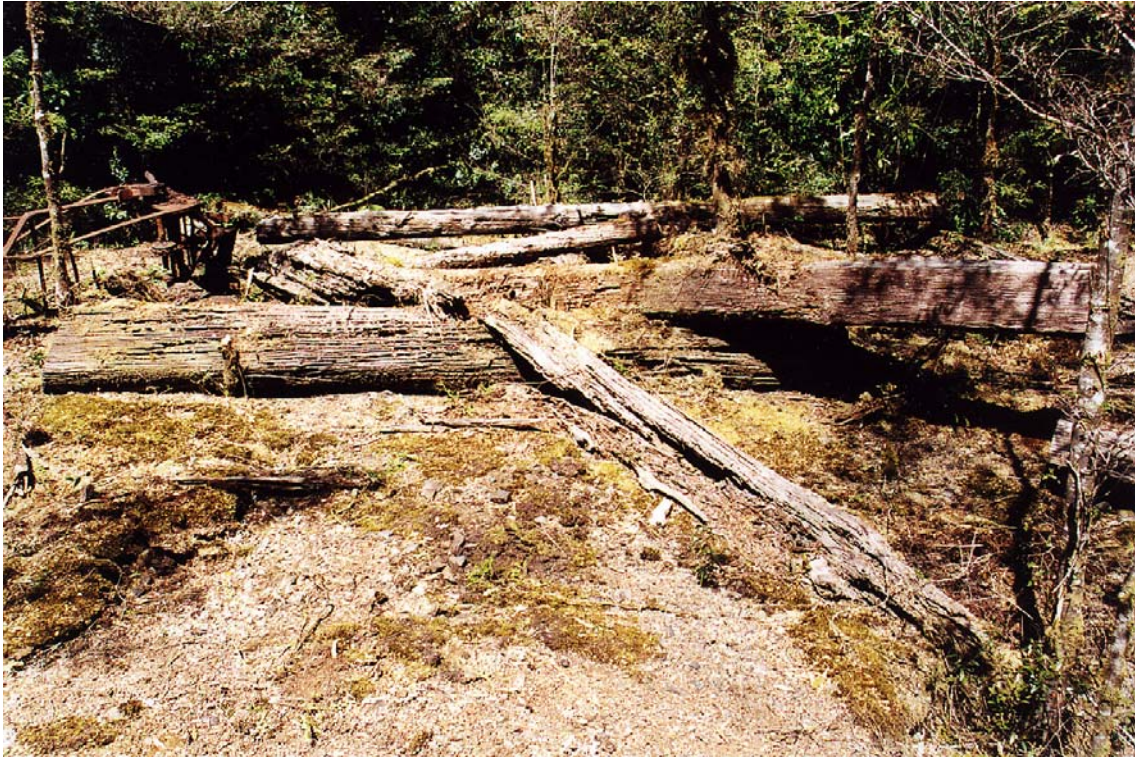
Ring Valley mine, view of collapsed headframe from main shaft
