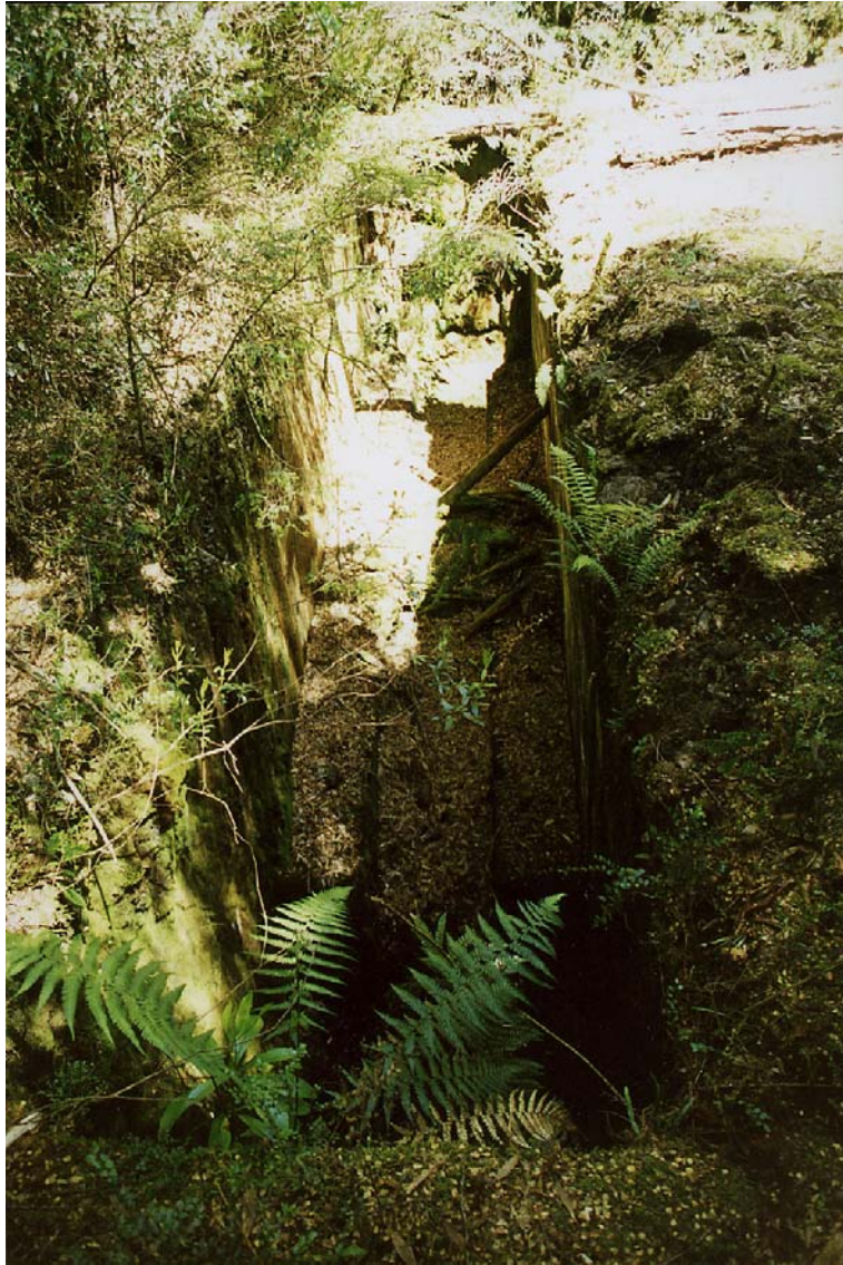
Ring Valley mine, view of concrete-lined pit used to accommodate the main shaft pumping machinery
