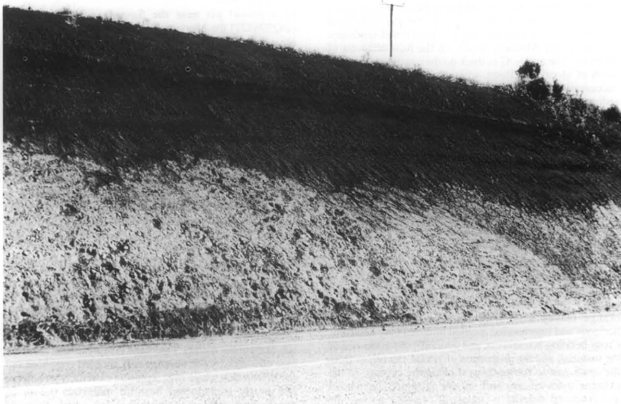
Plate 6. Weathered Thirlstane Basalt in a cutting on the Bass Highway.
