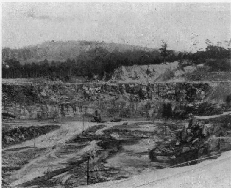
FIG. 23.—Goliath Portland Cement Co., Portion of Open-Cut.
