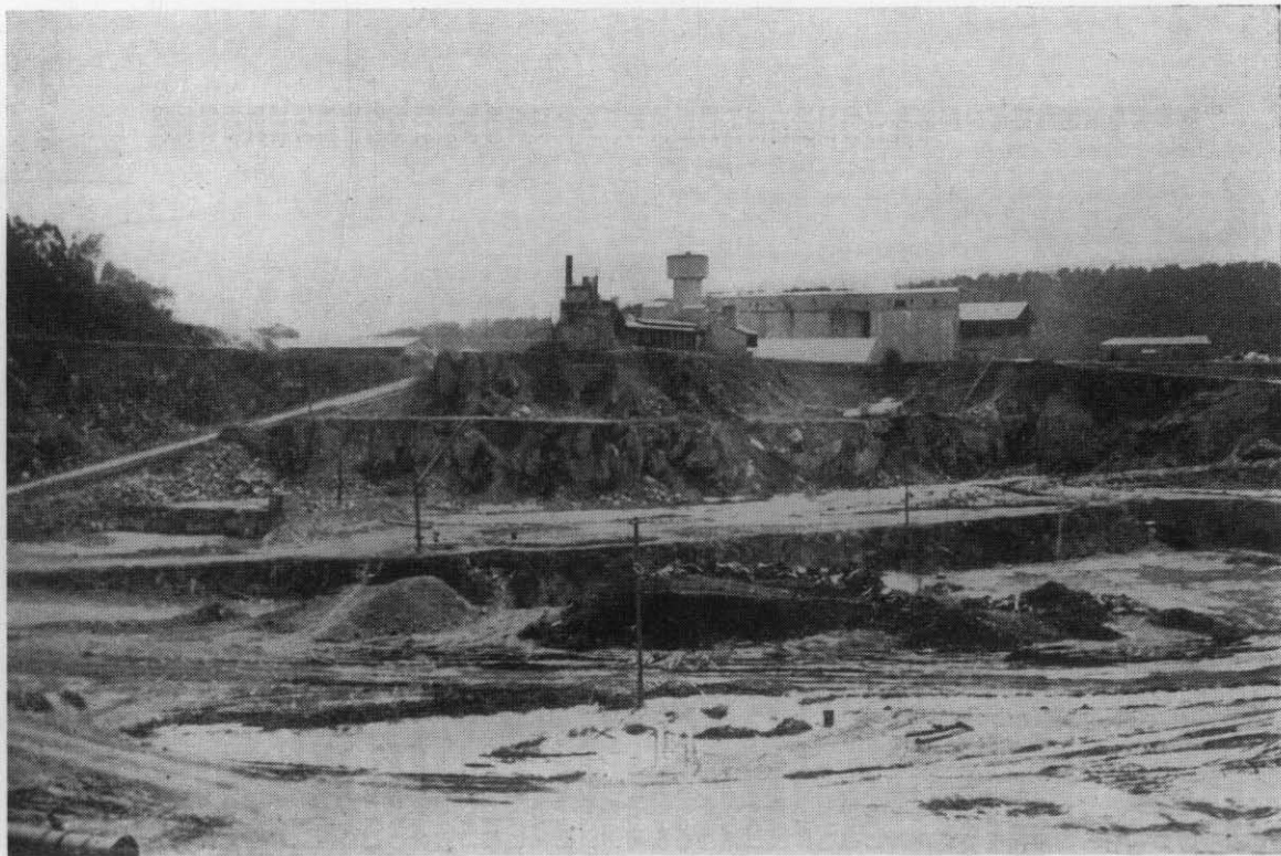
FIG. 1.—Goliath Portland Cement Co., Portion of Open-Cut and Works.
