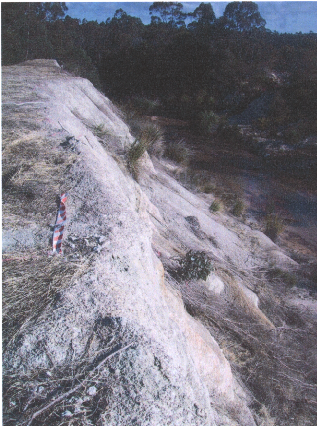
Left, Truncated spoil heaps with brush placed on steep slopes
