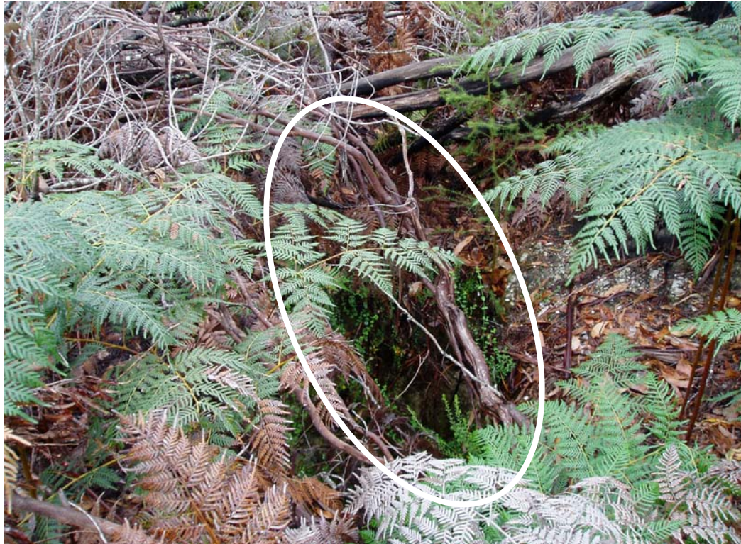
Figure 5. Example of an obscured shaft at the Union Mine. This shaft measures 2200 mm x 1200 mm and is open to a depth of 12 metres.
