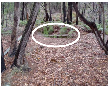
Figures 6 & 7. Two views of the Union Mine main shaft. This shaft is open to 11 metres and measures 3200 mm x 4200 mm at ground level. There are drives off the two long sides at the 11 metre level.
