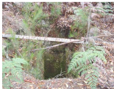
Figures 6 & 7. Two views of the Union Mine main shaft. This shaft is open to 11 metres and measures 3200 mm x 4200 mm at ground level. There are drives off the two long sides at the 11 metre level.
