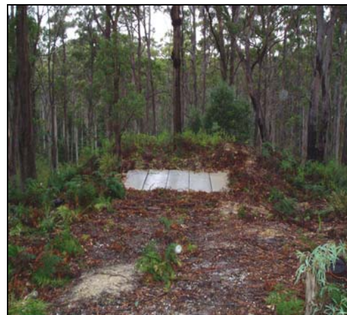
Figure 2. Gift Main Shaft. Covered with 5 x 3700 mm x 1000 mm panels.
