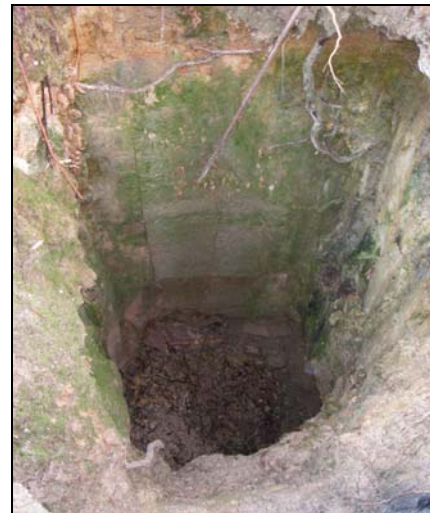
Figure 1. Shaft of the Monarch Mine. Fifteen metres off Forestry road — 2400 mm x 3600 mm and open to 12 metres with drive off right hand side.
