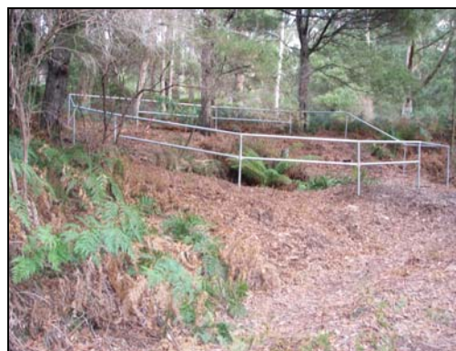
Figure 3. Work in progress on steel rail barrier enclosing the Volunteer Main Shaft.
