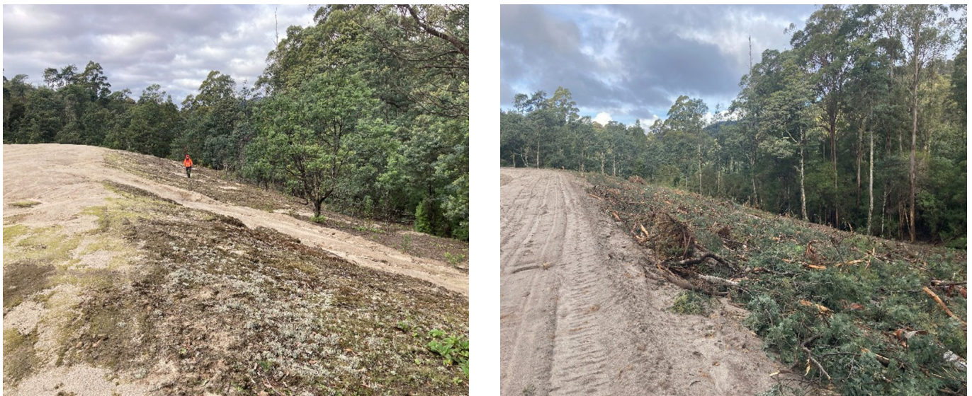
Figure 2. Comparison of Anchor embankment pre- (left) and post-remediation work (right).
