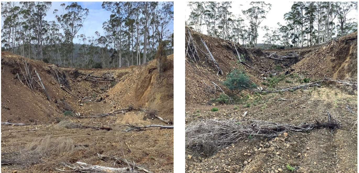
Figure 6. Comparison of site post remediation (2024) and recent inspection (2025).
