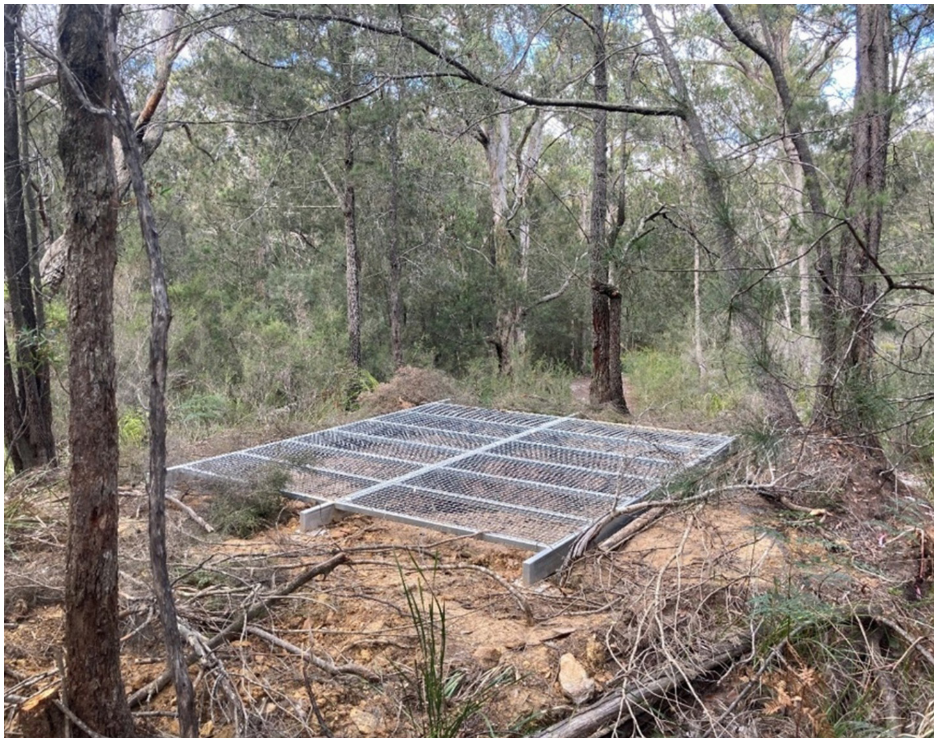
Figure 21. Fabricated cap installed at Equilla Site (April 2026).
