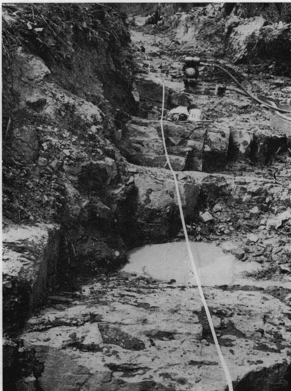
PLATE 1. Trench between cut-off wall position and dam site centre line, Whitewater Creek.
