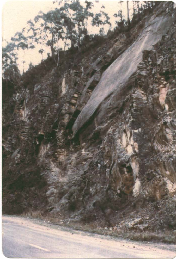
Plate 5. Planar failure along the bedding plane on an upper limb of a fold.
