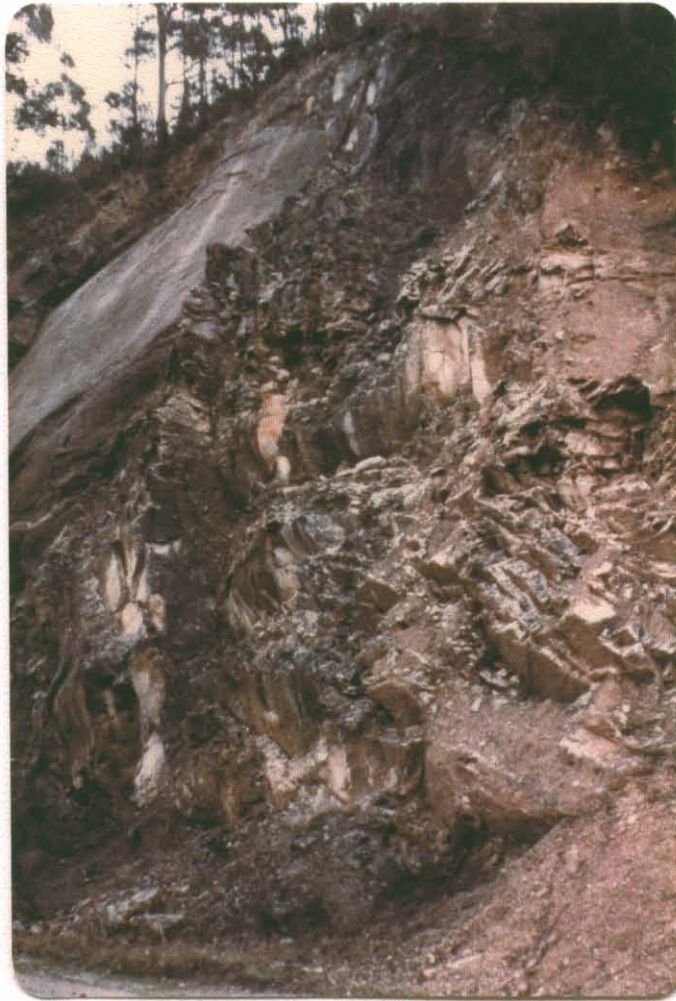
Plate 13. Bedding with a component of dip towards face resulting in a lower face slope angle, and instability leading to wedge and planar failures.
