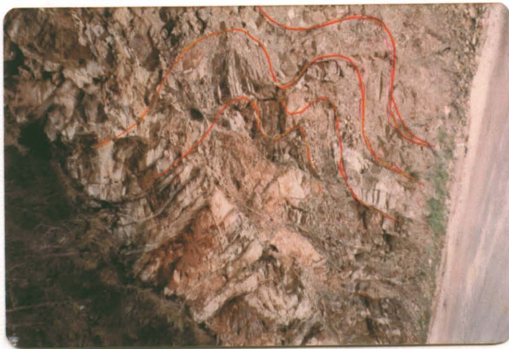
Plate 11. Style of folding in the argillite showing complex wedge failure in the contorted and crushed zone in the nose of a fold.
