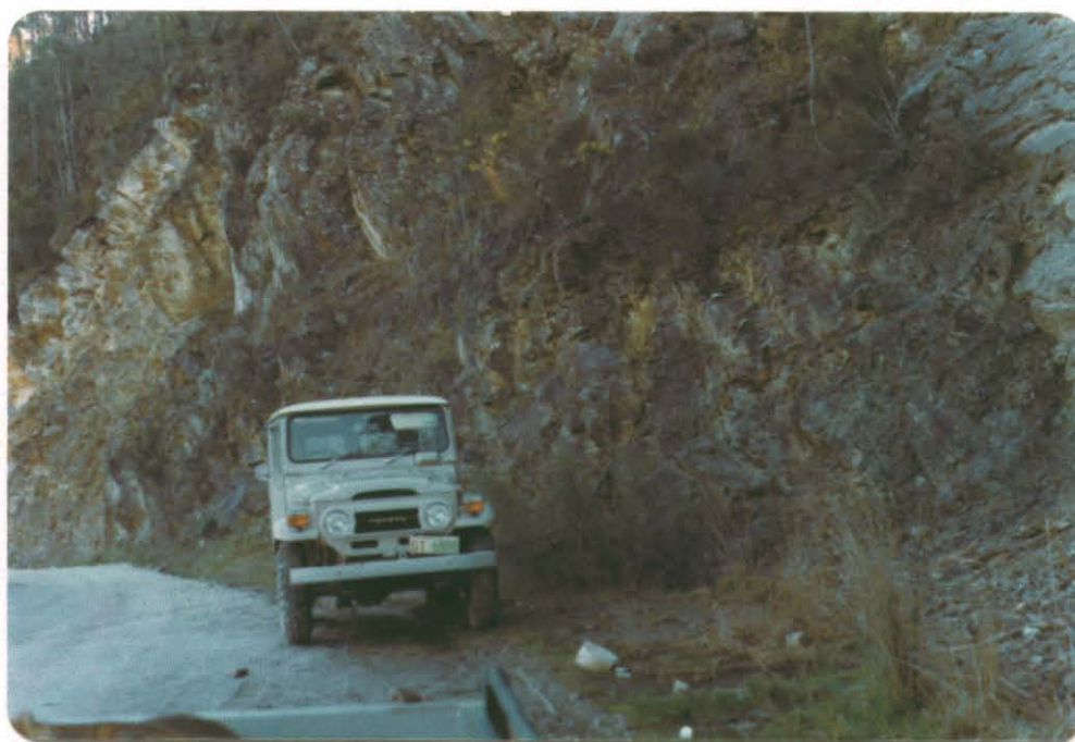
Plate 12. High face angle and local stability due to the bedding having a dip component away from the cliff-face.
