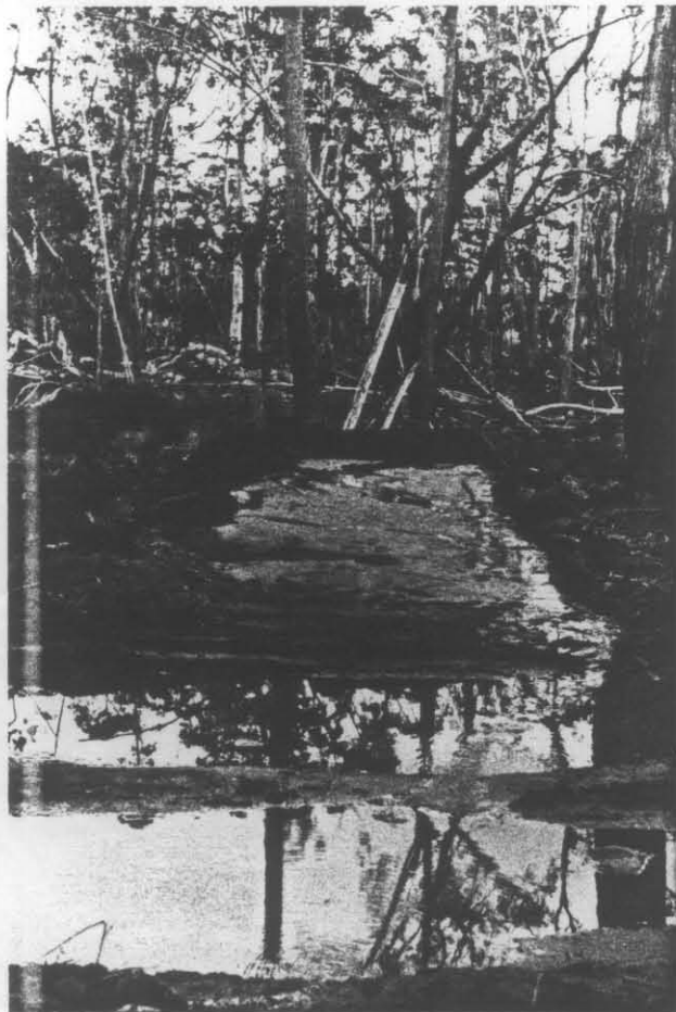
Plate 2. 'Scoop' or roadside push-off area (Central Highlands) in an area of easily eroded windblown sand. 'Scoop' acts as settling pond providing a good sediment trap.
