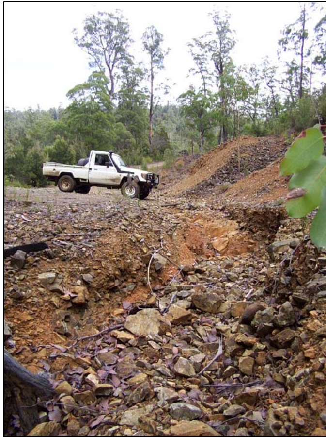
Plate 6: Washout on Forestry Track (5412360N, 361640E).
