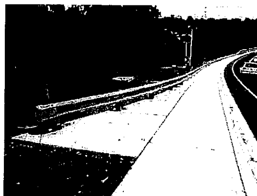
Figure 23: Slotted breakaway cable terminal (SBCT)
