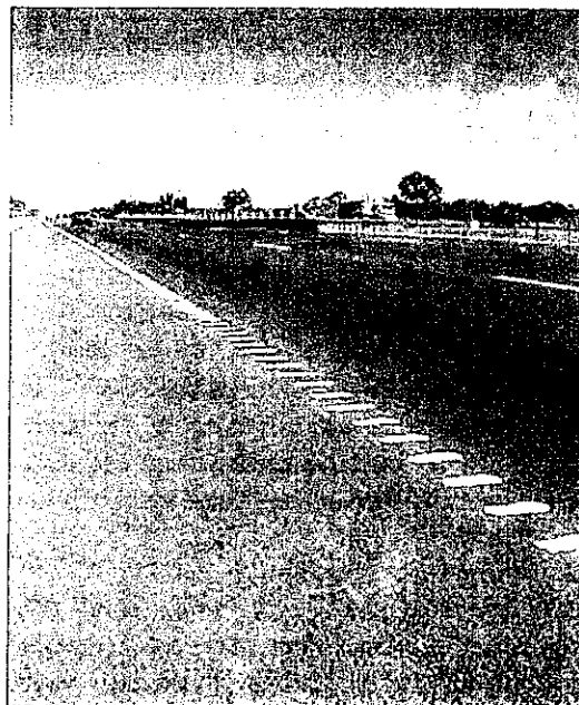
Figure 1: Audiotactile edge lines on a freeway
