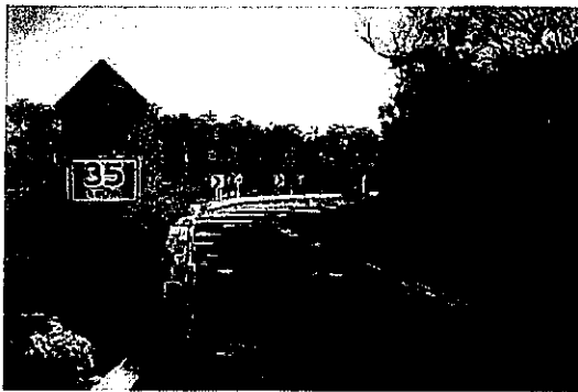
Figure 3: Warning sign, advisory speed sign and chevron alignment markers (CAMs) at a sub standard curve
