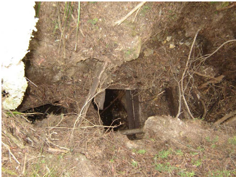
Plate 3: Three compartment mine shaft in western portion of study area.
