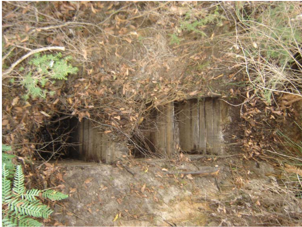
Plate 3: Three compartment mine shaft in western portion of study area.
