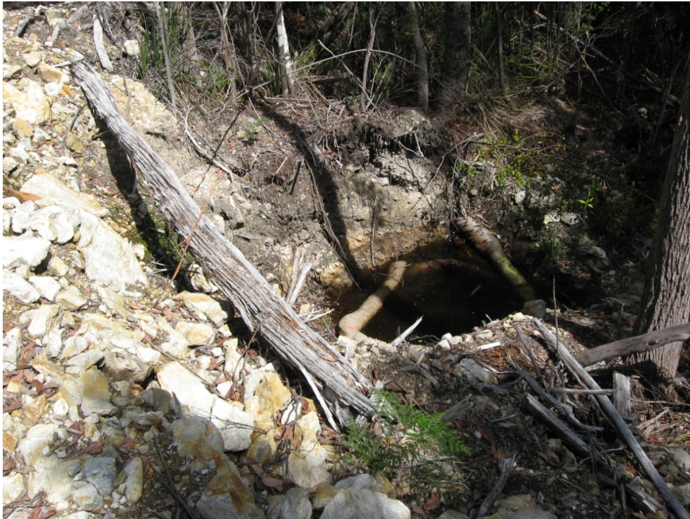
Sump off edge of BHD-9 pad needing filling and contouring
