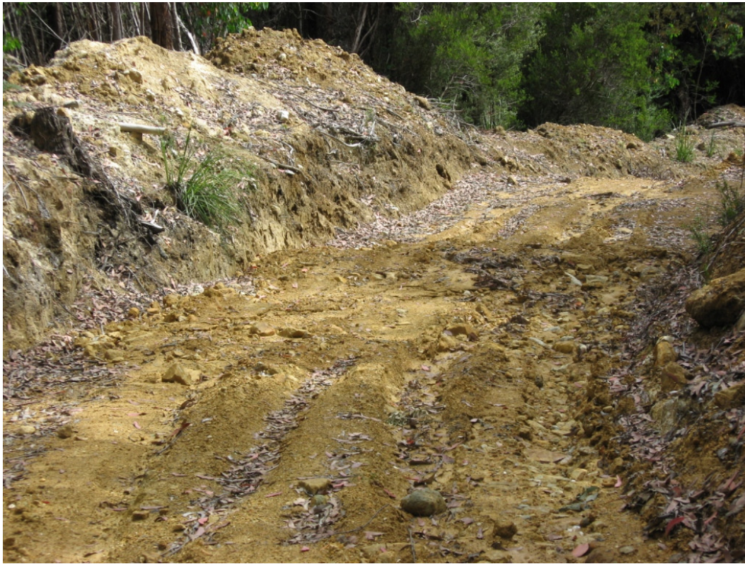
Main Sock Creek track to BHD-7 – note drainage across track
