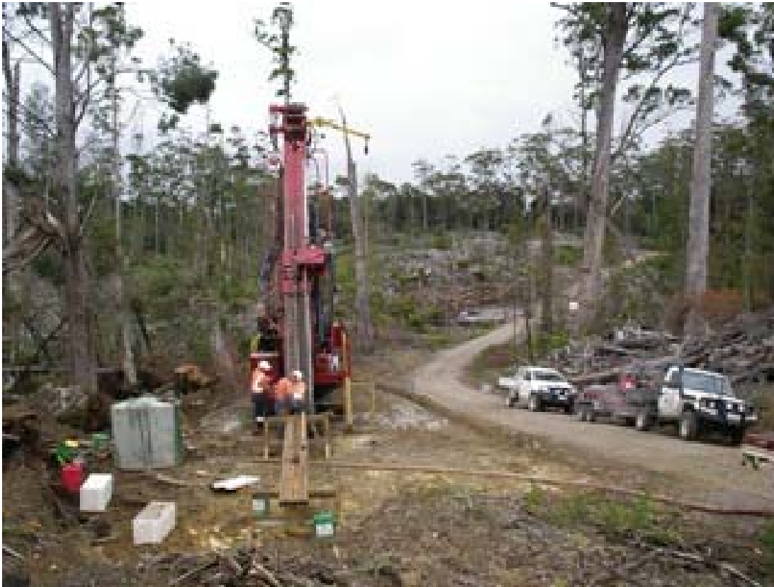
Figure 3. Drillrig at Dunns
