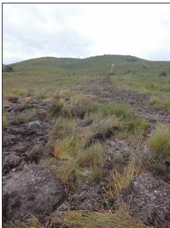
Main Access Track - Rehabilitated
