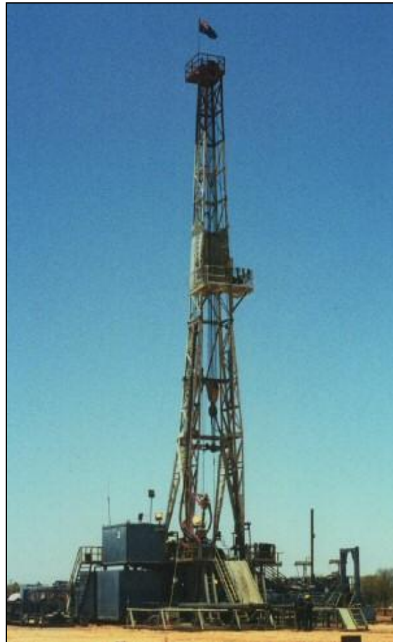
Figure 7: Hunt Energy Rig 3 at Westwood #1 Location
