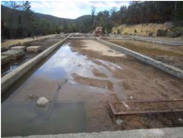
Plate 3 NGG battery site with 1980's overprint : Photo ref
