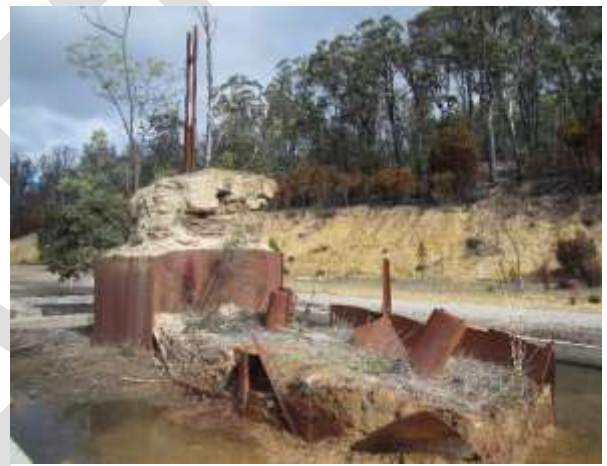
Plate 4 1980's Tailings Retreatment : Photo ref
