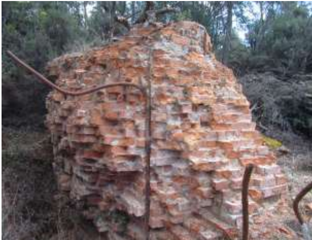
Plate 1 Winder foundation : Photo ref 1-4
