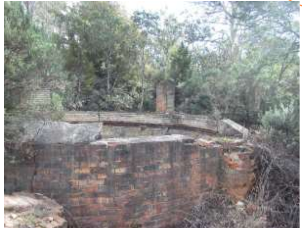
Plate 2 NGG Tanks : Photo ref 1-4
