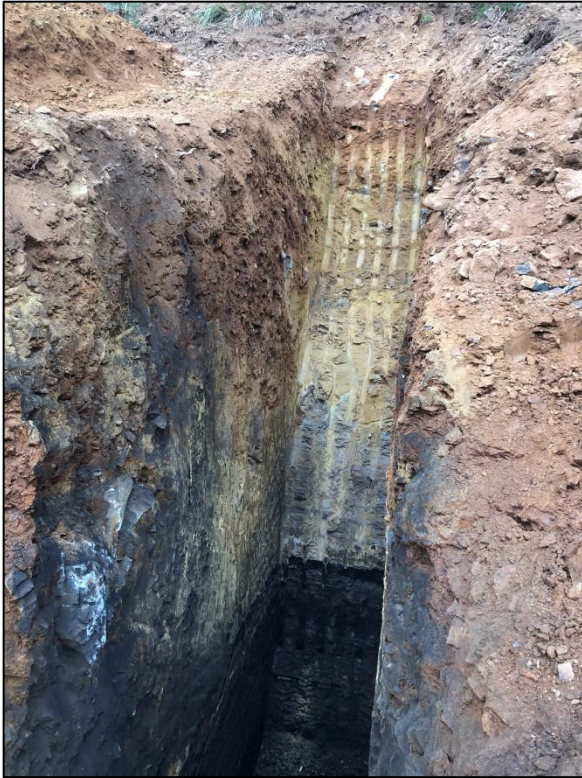
"B" Headings Portal Trench
