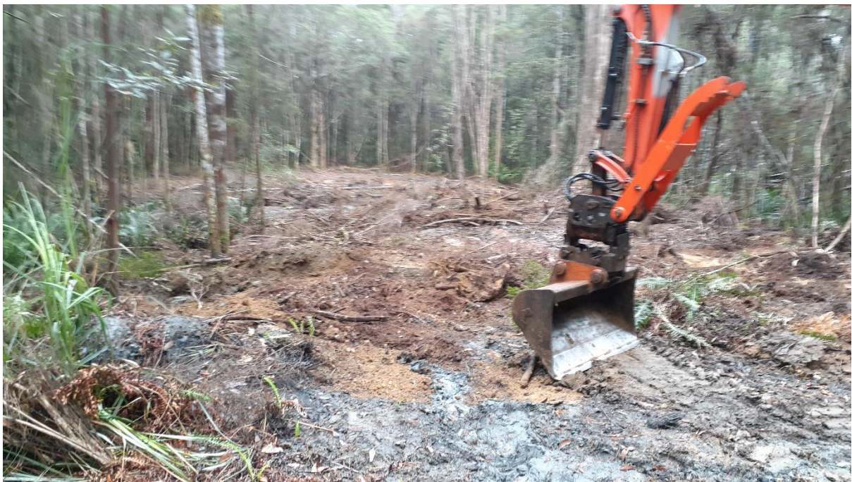
Figure 7. MF112/113 drill pad after rehabilitation with excavator. Loose vegetation has been used to cover the area to promote regeneration.
