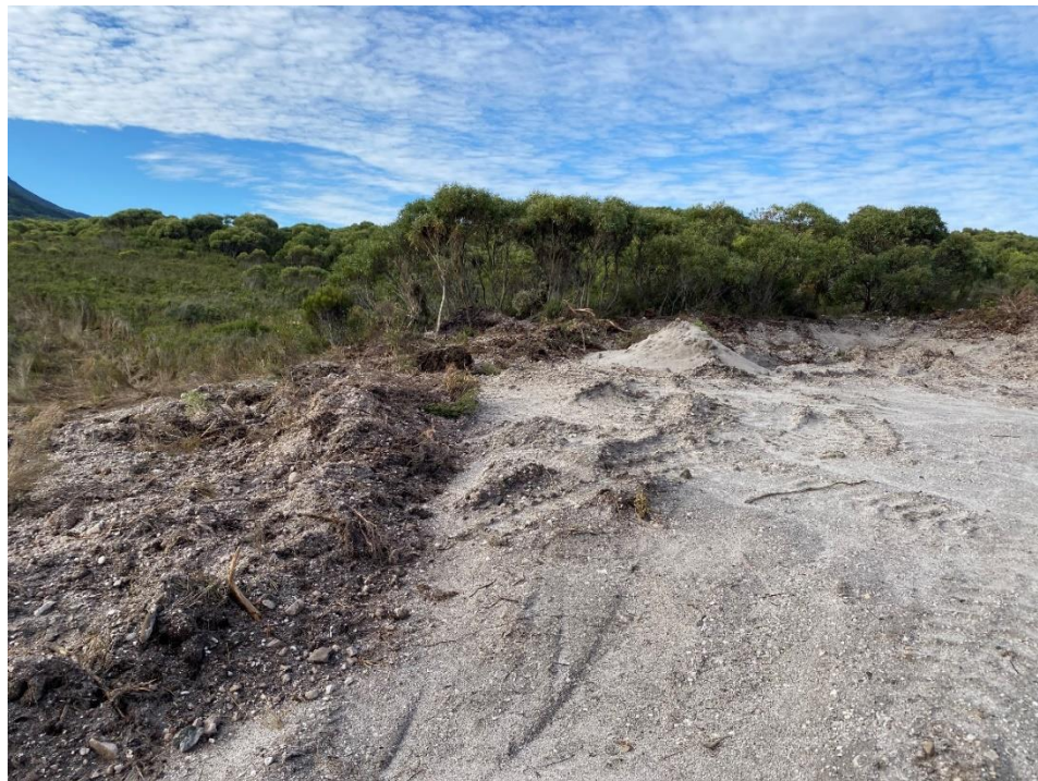
Figure 6. Rehabilitated Denali drill pad with ground levelled and collars buried.
