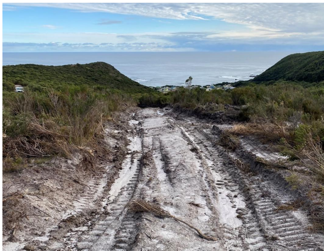
Figure 8. Top: Drill pad levelled with sumps filled. Bottom: Repaired four-wheel drive track.
