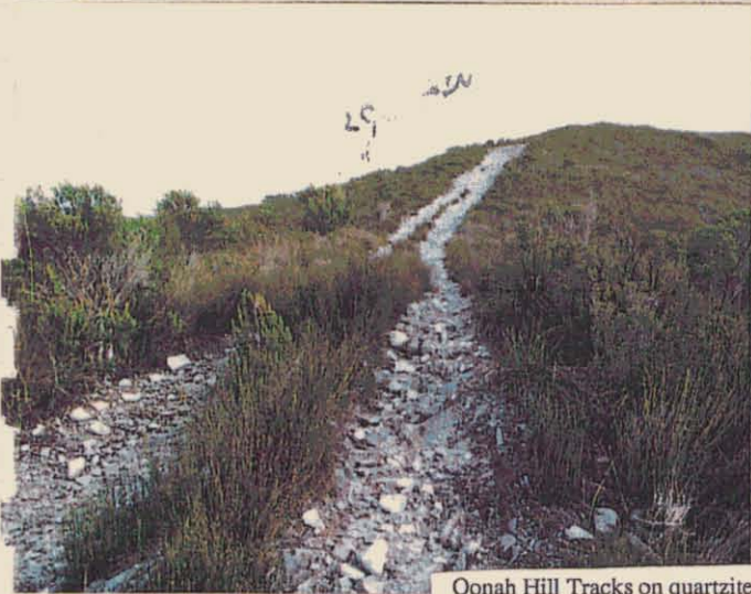
Oonah Hill Tracks on quartzite and in rainforest Tracks to be closed, ripped and gripped, soil returned from edges and revegetated.
