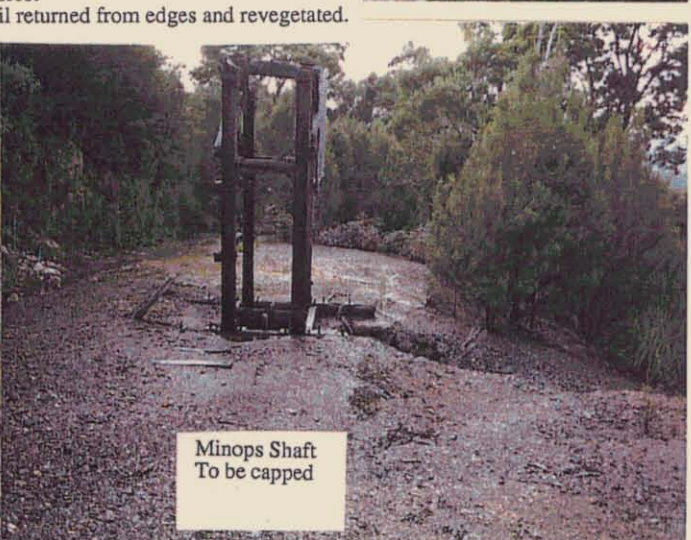
Oonah Hill Tracks on quartzite and in rainforest Tracks to be closed, ripped and gripped, soil returned from edges and revegetated.
